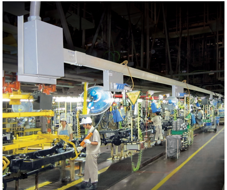
Continuous open-channel busway with easily modified circuits
